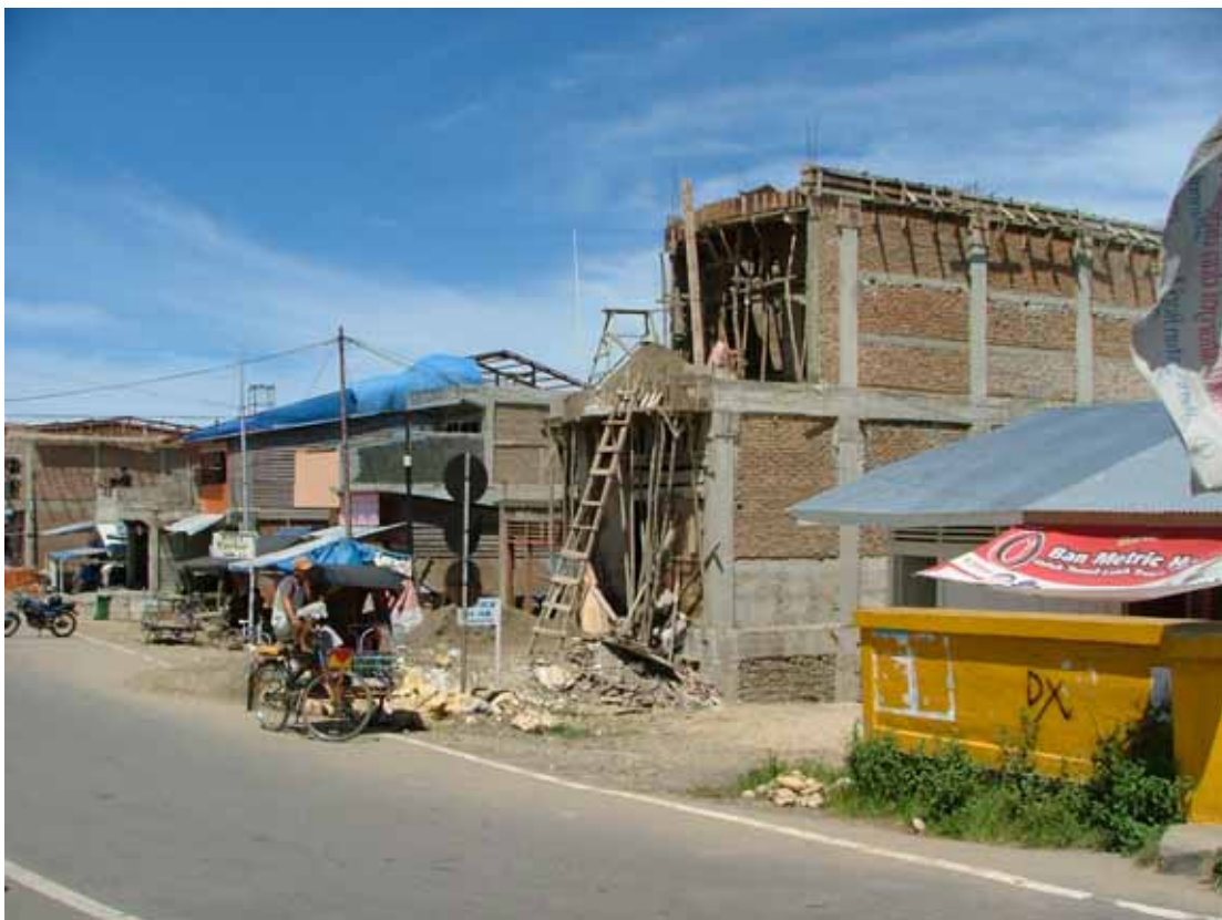
At the northern end of the bridge above, all the original buildings were flattened by the earthquake. The rubble waste-land is now transformed by these new, well constructed buildings.
